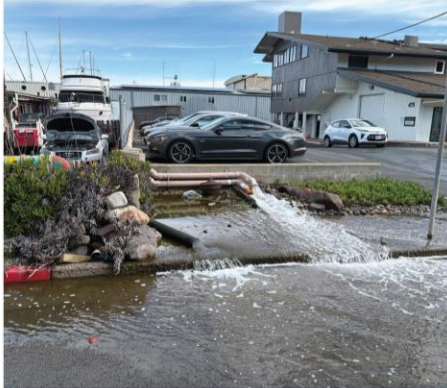
Private property pumps discharge onto Gate 5 Road
