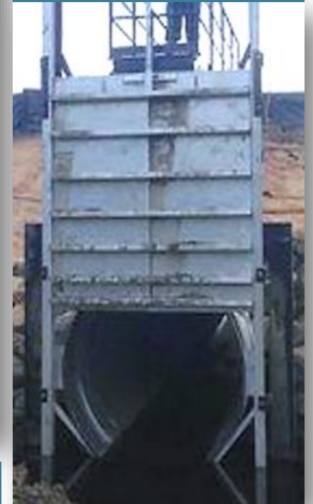
Tide Gate – Automatic, Vertically Operated Sluice Gate
