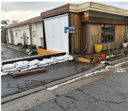
Sand bag protection on Gate 5 Road
